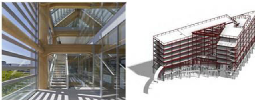
Figure 11.2 Tamedia Office Building Zurich, Switzerland. ( Source: Google Images)
